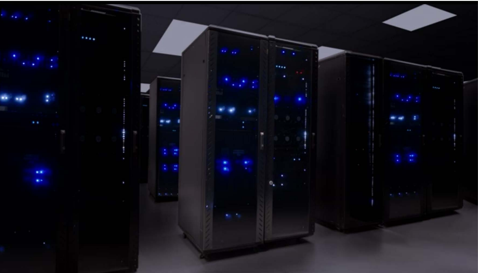
FIG 1 – Screen grabs of Lakeview Data Centre and server room ( Upload , 2020).
